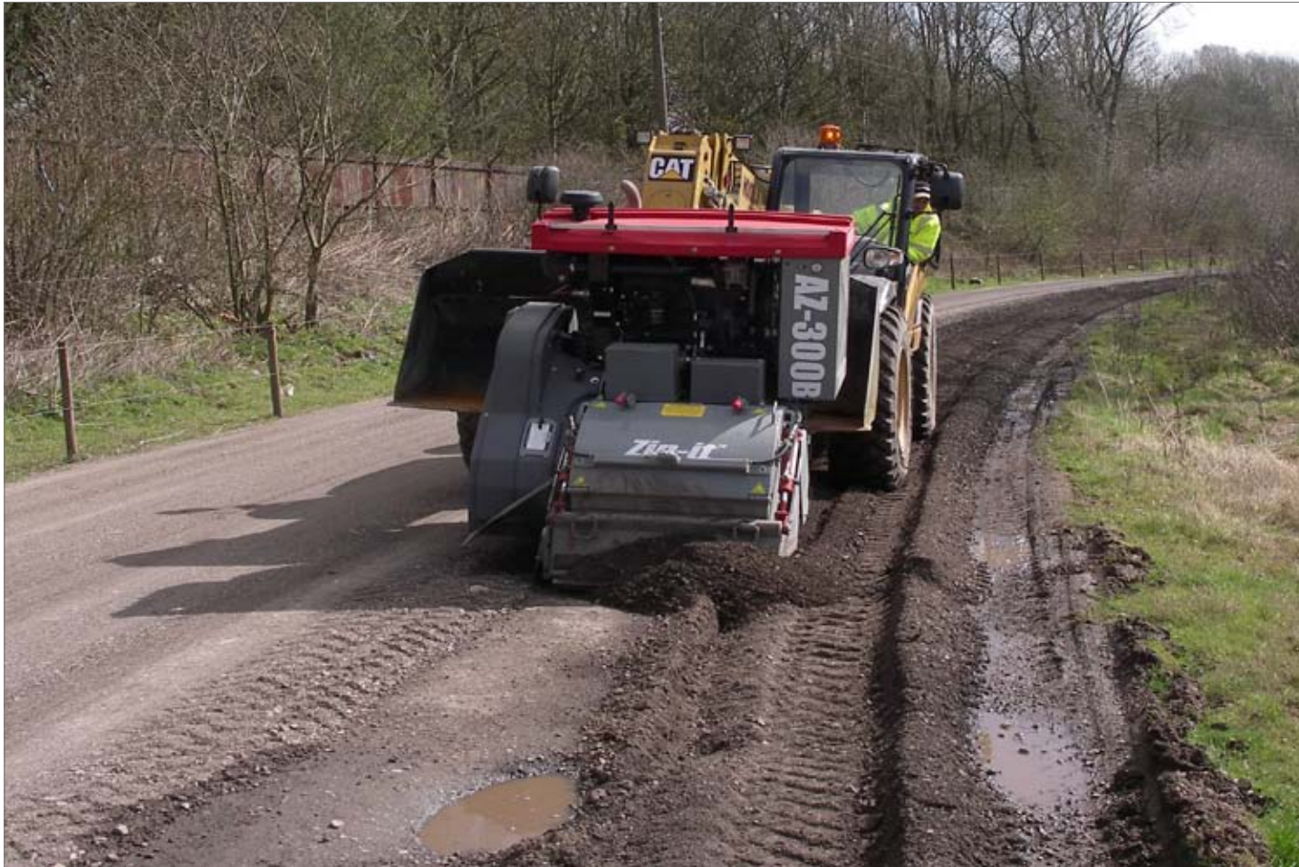
After milling and rolling
