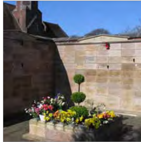
Cremated Remains Niche System Installation - South East London
