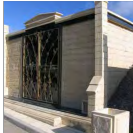
Embankment Mausolea Installations - North London
