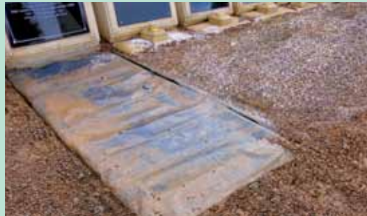
The final cover slabs are protected with plastic sheeting.
