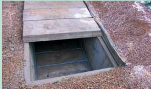
Each level is hermetically sealed using water resistant resins.
