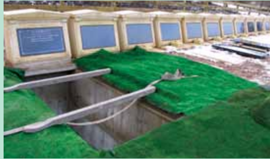
Chambers provide clean and safe burial facilities in all weathers.
